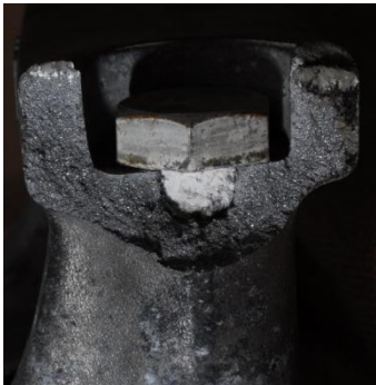
Figure 18: Typical Cleat Fracture
