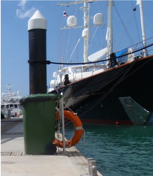
Figure 9: Steel Pile used for mooring.
