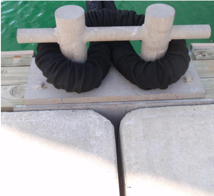
Figure 13: Bollard mounted through two concrete pontoons
