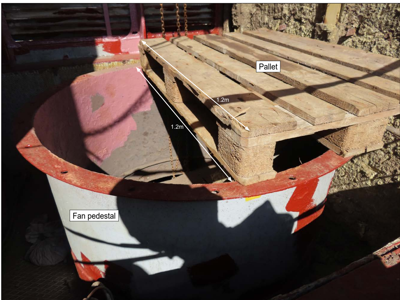
Figure 10: Pallet on the fan pedestal in the position it was reported to have been found
