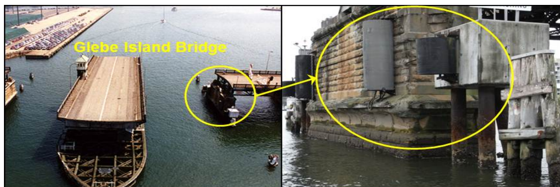
Figure 8: Glebe Island Bridge structure and fenders
