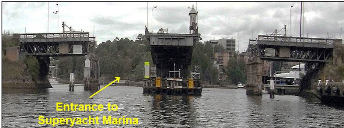
Figure 3: Glebe Island Bridge opening
